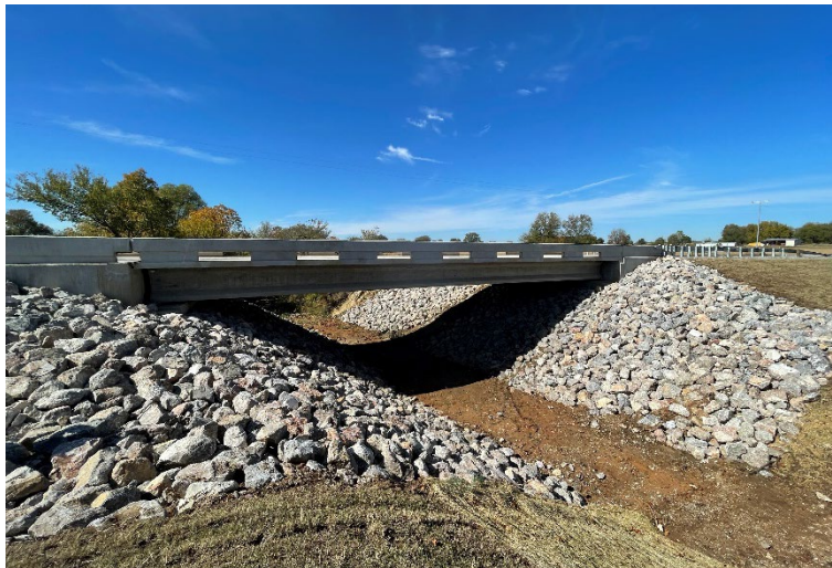
Tributary to Chigley Sandy Creek, Murray County
